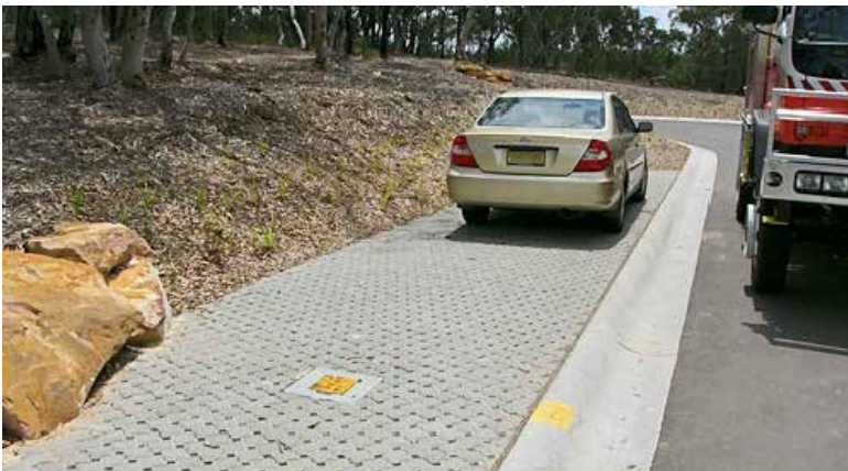
Figure 15. Hydrants and parking bays.
